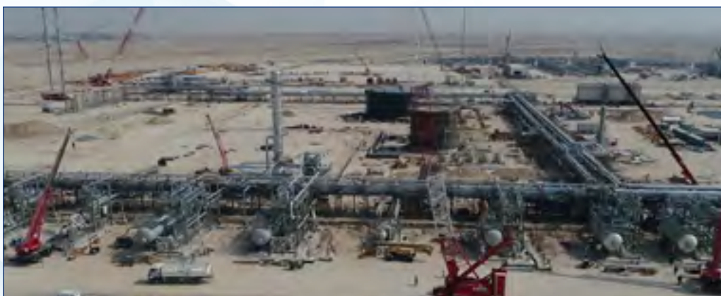
CONSTRUCTION PHASE OF COMPLETE OIL TRAIN
